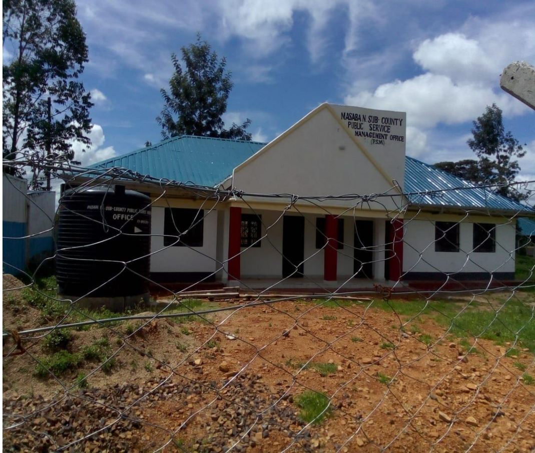
Completed Masaba North sub County offices
