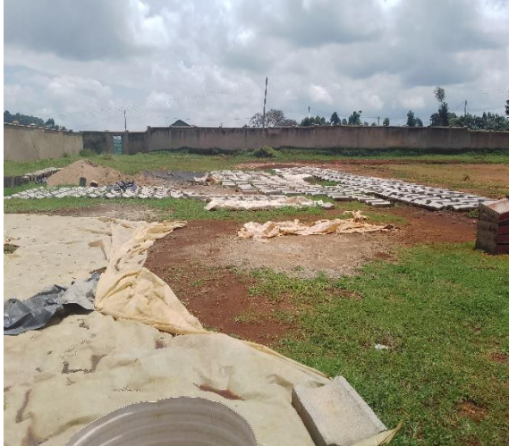
Drainage works Manga stadium
