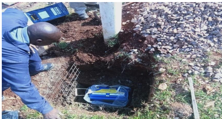
Repair of streetlight at Magwangwa market
