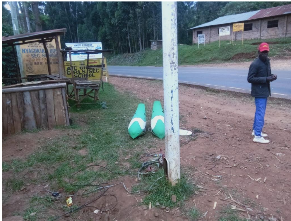
Repair of Nyagokiani junction streetlight
