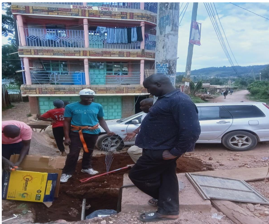
Repair of Keroka Market streetlights - Roy Resort Gate
