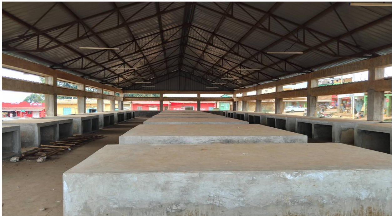
Completed phase 2 construction of Nyabite market shed.
