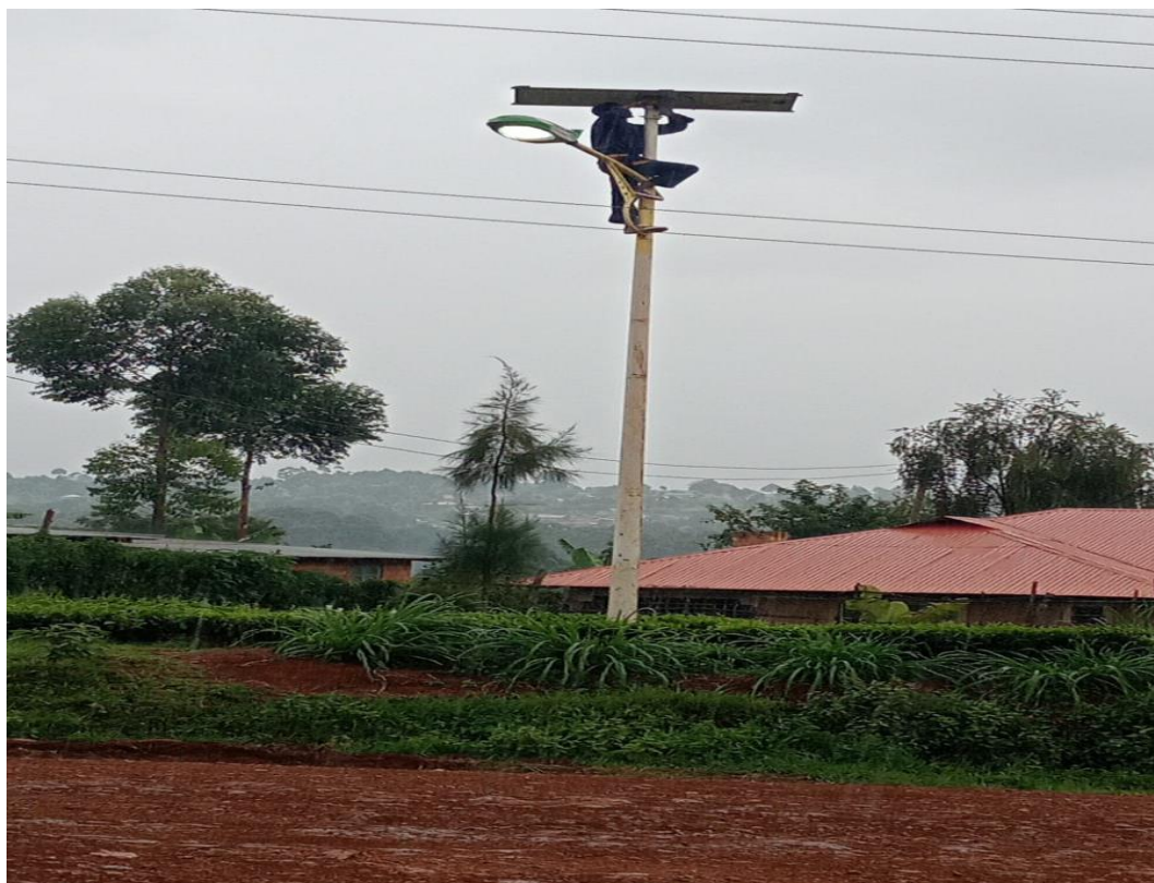
Marindi-Kenyorora junction repair works
