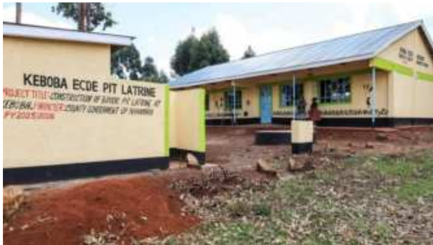
Figure 5 complete classroom and a two door pit latrine
