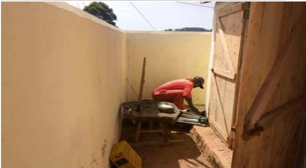
TING'A MARKET SHED (Installation of grills all round with 4 lockable door, replacement of missing cubicle doors, paint work, floor repair, water connection to existing 5000L tank.)
