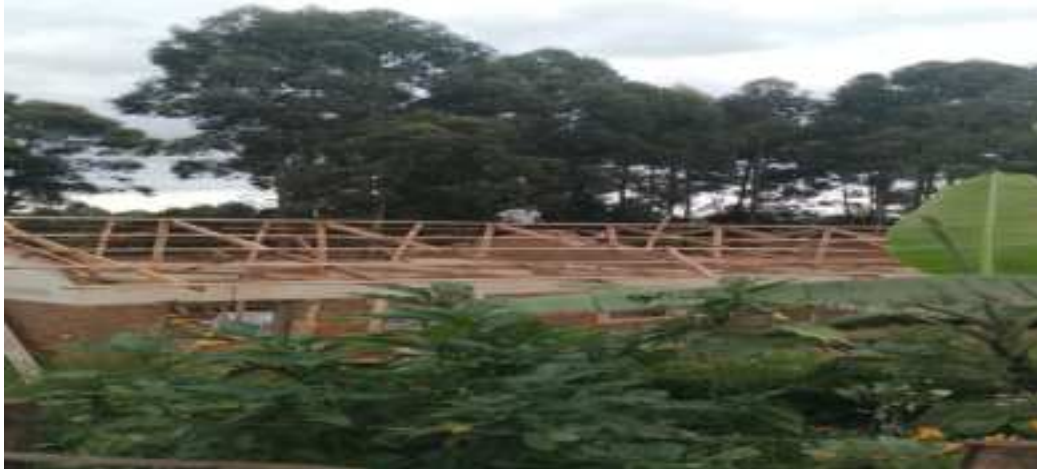
Figure1 Renovation of the roof
