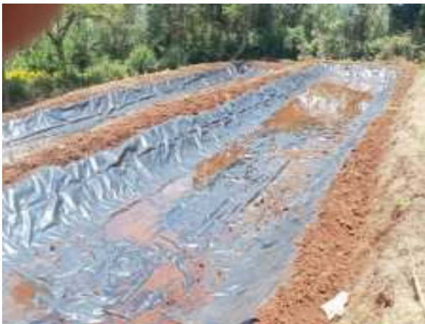
Picture 1.3 Kareha Investments Ltd's Matutu Farm two of the eleven [11] fish ponds fitted with pond liners and a water pan supervised by Borabu fisheries team.
