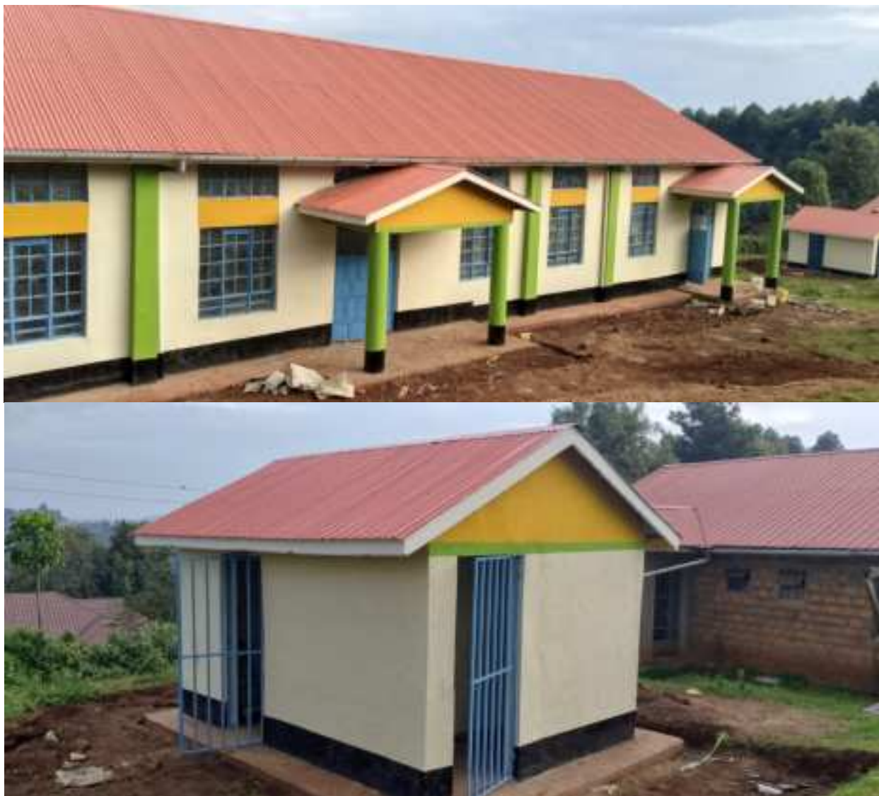
Completion of Social hall and abolition block at Keroka
