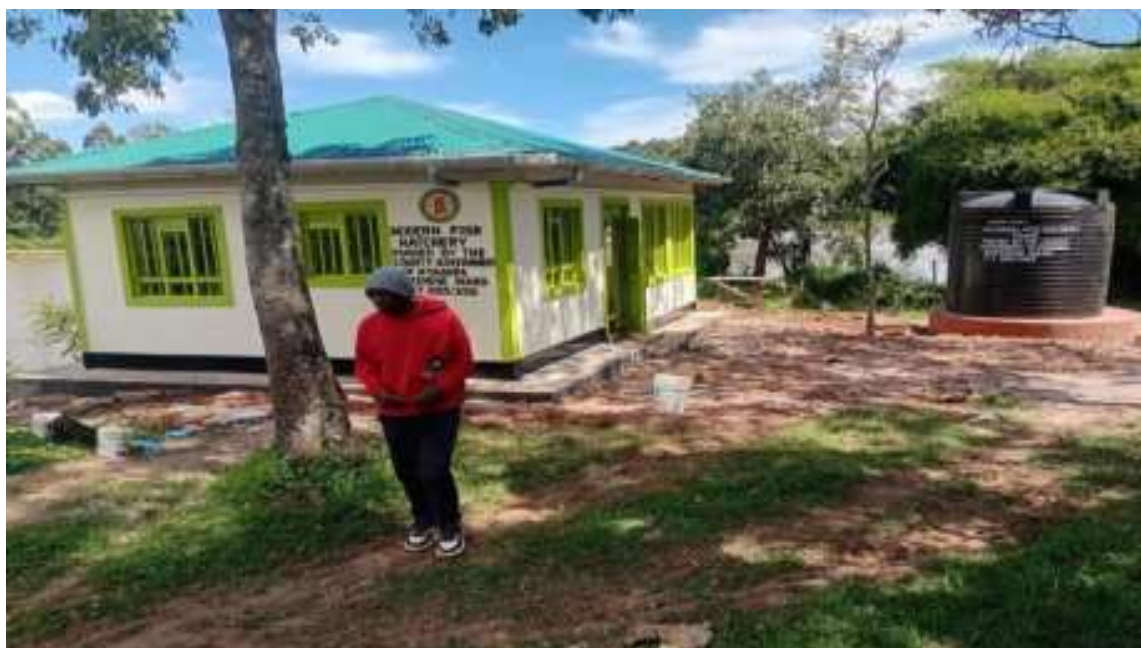
Figure 3: showing county fish hatchery with a 10,000litre tank in place with paint works, signage & branding also done.
