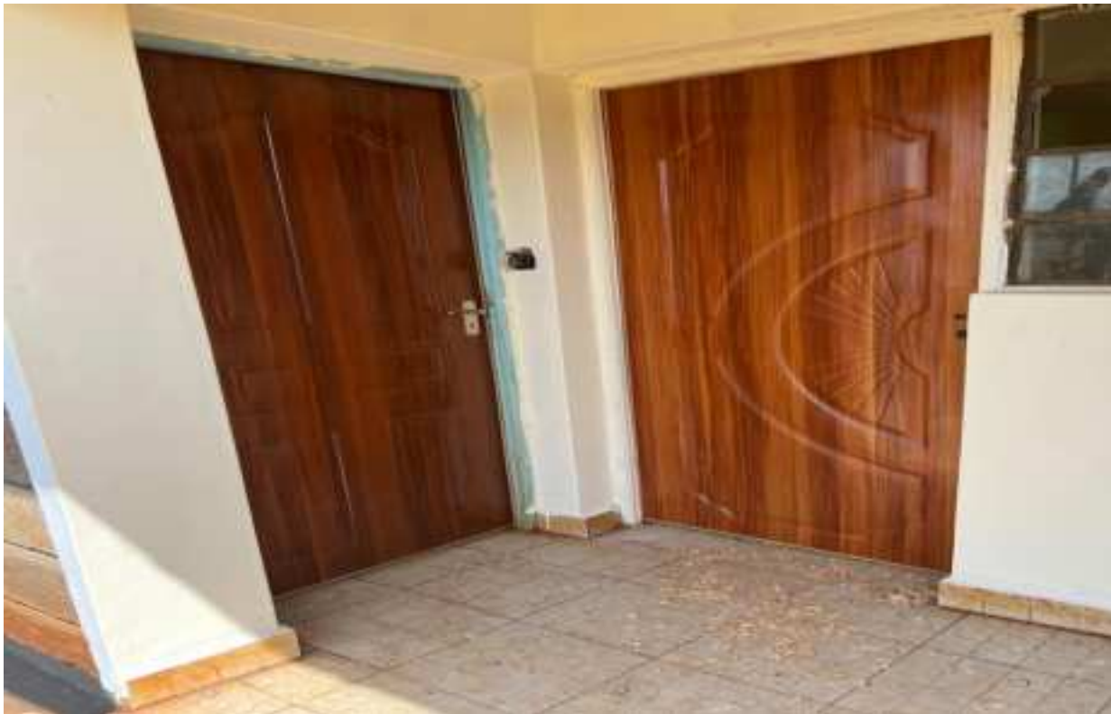
MAGWAGWA MARKET (Renovation of market shed roof, rainwater storage tanks, toilet, chain-link fence & gates.)
