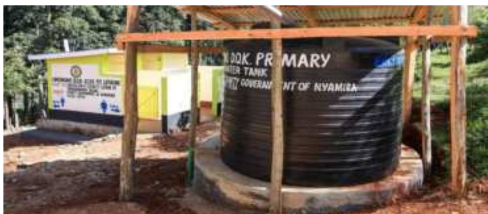
Figure 7 Complete classroom. 5000 litres tank and two door pit latrines
