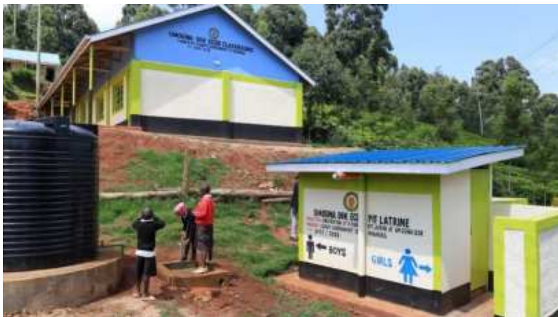
Figure 6 Complete classroom. 5000 litres tank and two door pit latrine
