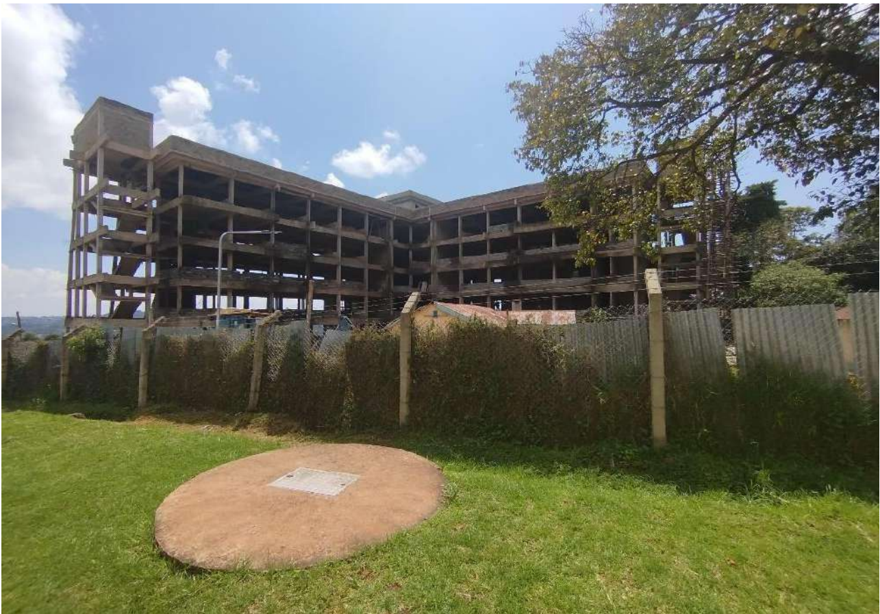
Ongoing construction of county headquarters
