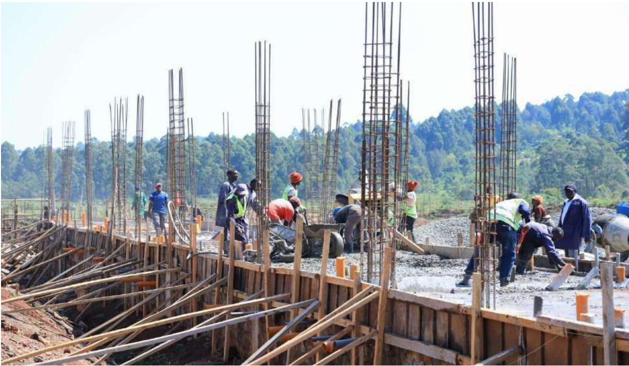
Construction of 8 units at Sironga industrial park
