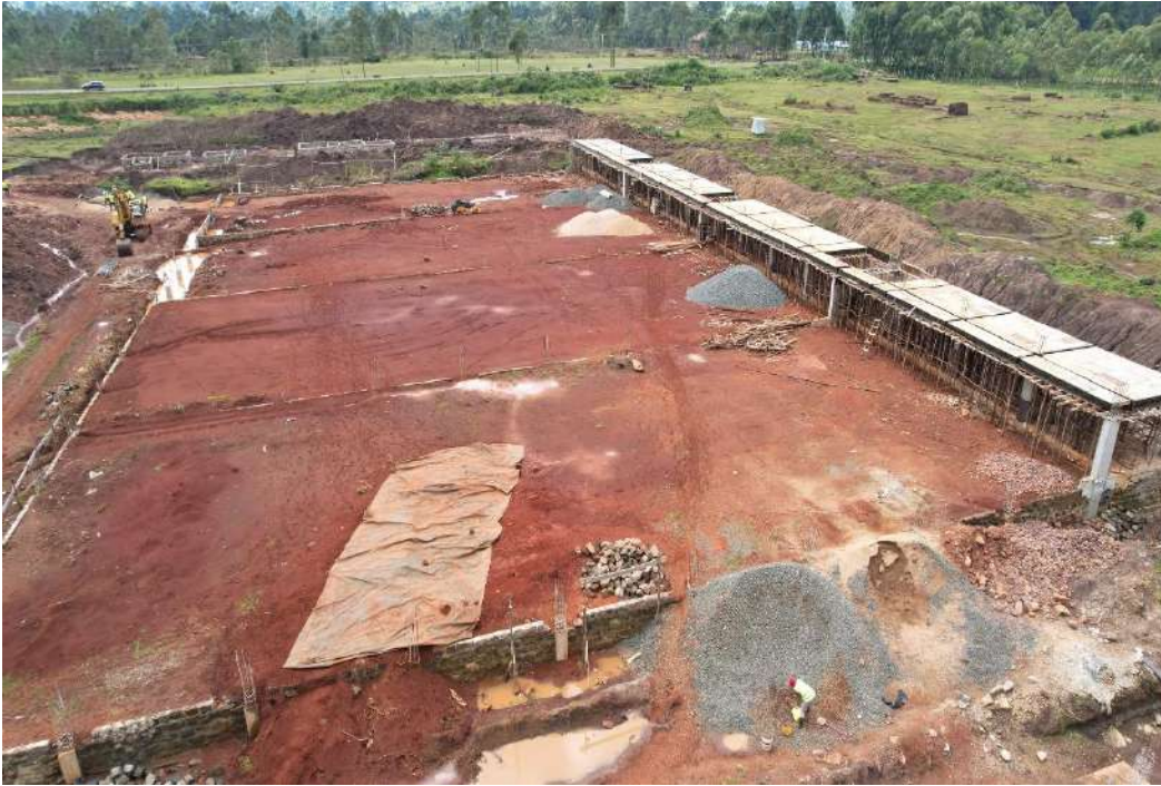
On-going construction of 8 units at Sironga industrial park
